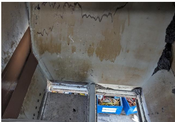
Figure 7: Hopper Interior (Before)
