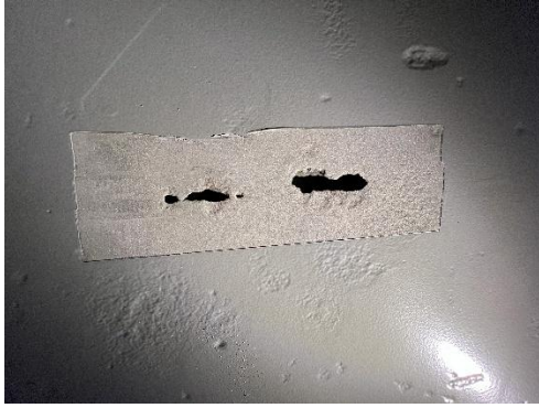
Figure 3: Penetrations in hopper wall
