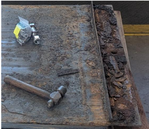
Figure 2: Corroded slide gate
