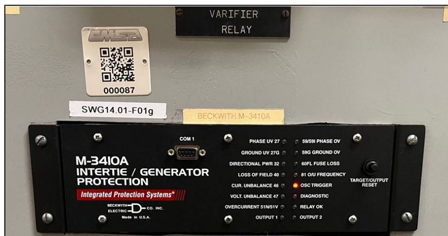
New switchgear relay installed
