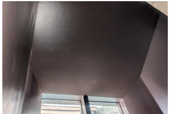
Figure 8: Hopper Interior (After)
