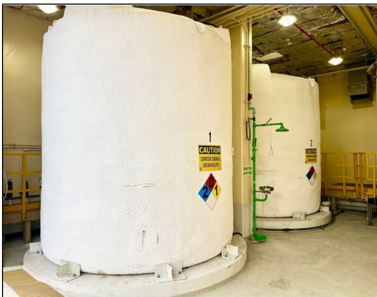
Two new SBS tanks installed
